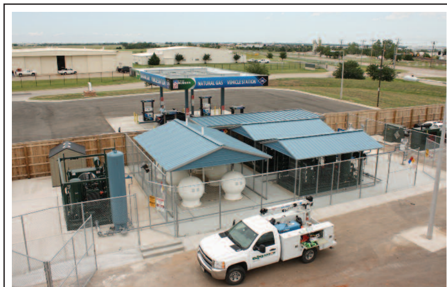
This natural gas fueling station is one of 10 that uses compressors made by Arrow Engine Co. Arrow reports that inquiries about its CNG compressors, which use a vibration-minimizing design, have become more frequent as fleets’ interest in the fuel grows.
